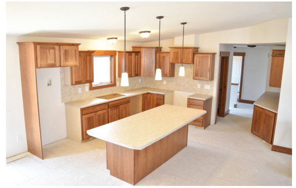
Under construction standard kitchen shown (sink missing).
